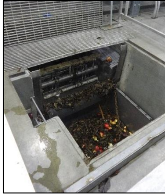
Product cull drains provide ample moisture and nutrients for Listeria, and should be well maintained to avoid back-ups or other routes of environmental contamination.
