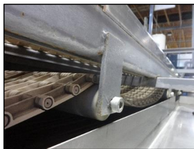
Underside of conveyors
