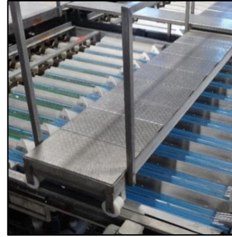
Extra care should be taken when cleaning platforms above product lines, especially if niches exist where Listeria may be able to harbor, and subsequently be 'squeezed' out by the weight of an employee
