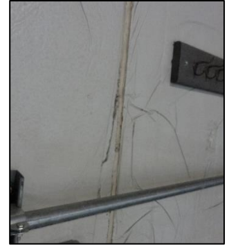
Cracked and caulked walls are common harborage points for Listeria
